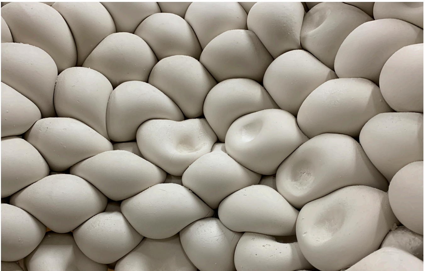
Figure 10. Interior of the inclined curved wall structure.
